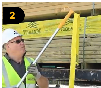
2 Lift the strap using the ProPole with ProHook attachment
