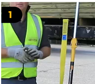
1 Secure the end of the tail strap to the lashing point
